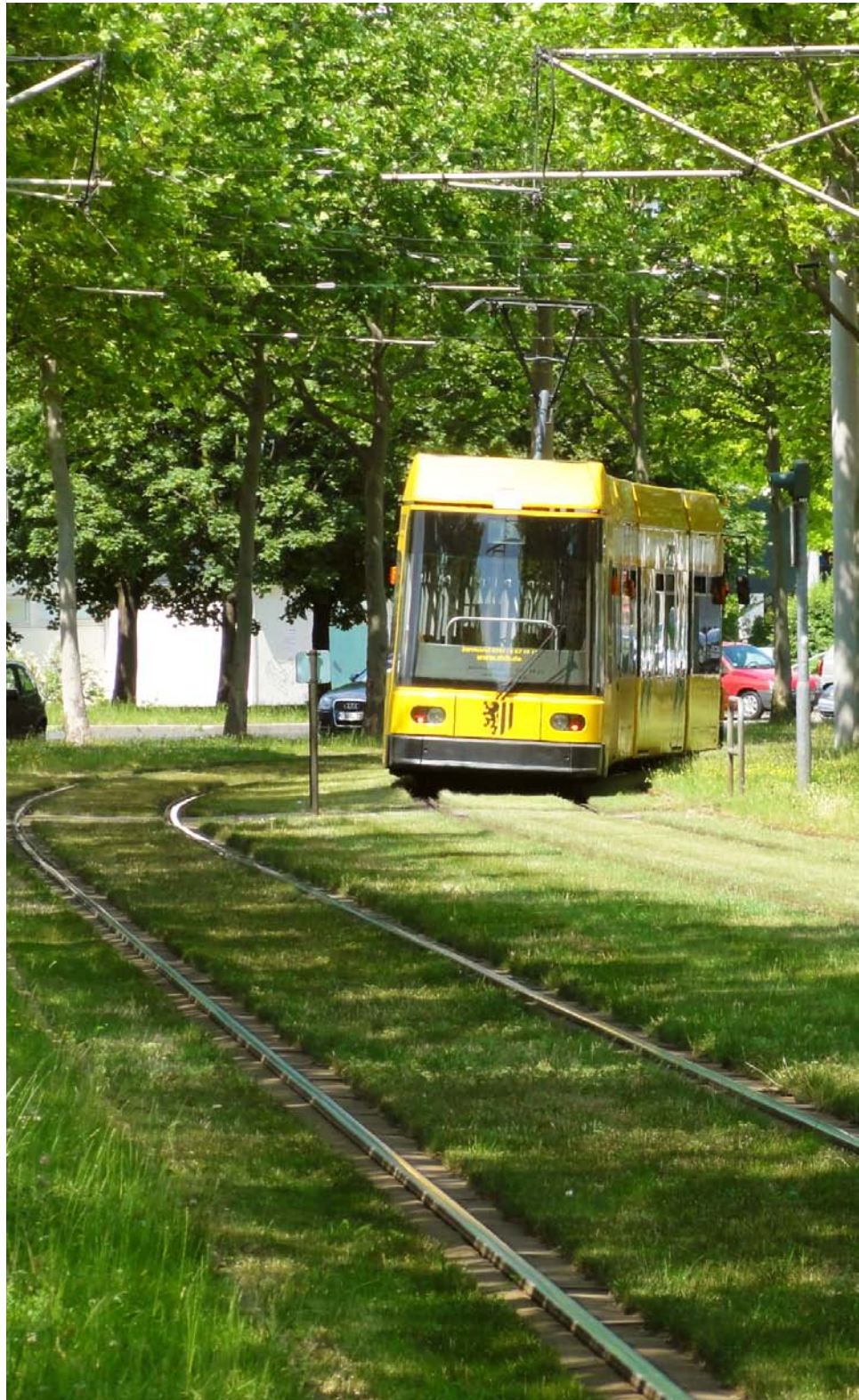
↓ Green tram tracks: improving the city's landscape and climate (part of line 13 in Prohlis)
